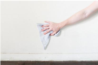
2. Make sure the wall is flat, clean and that all dust is wiped away. Fill any gaps in existing plasterboard with acoustic sealant.
