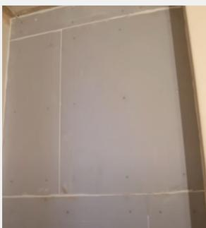
7. Start the second row from where the first ended to give the boards a staggered joint. Follow the same procedure until the wall is completed. Ensuring the first board is flush and square will make the rest of the installation easier.
