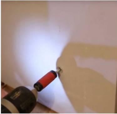
5. While holding the boards in position use suitable length drywall screws to fix the board into the stud work. Screws should go into the stud at least 25mm. We recommend a screw every 200 - 300mm on each vertical stud. The screw head should be flush with board when screwed in place.
